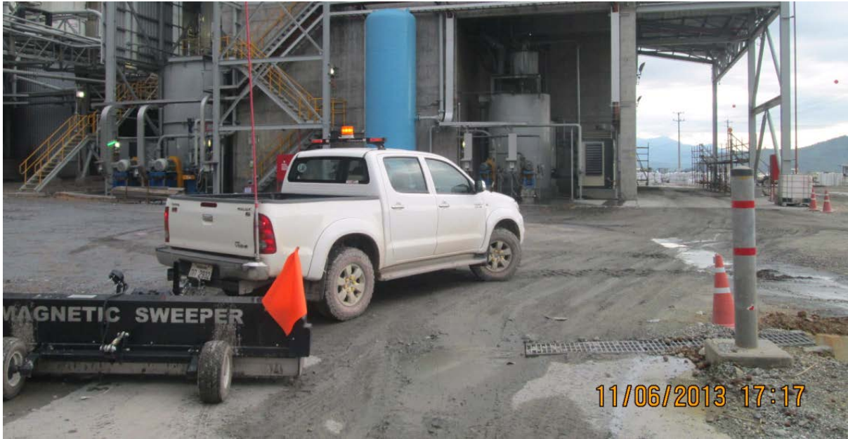
Found Scrap grinding media ball and other wire etc.. (Between 2 Shed )
