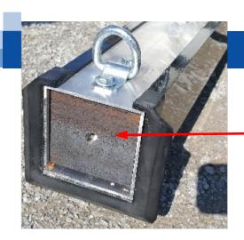
An Aluminum end cap (Part A from the cardboard box) needs to be installed over top of this internal steel end cap. (shown in next step)
